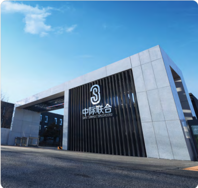
Headquarters in Beijing
